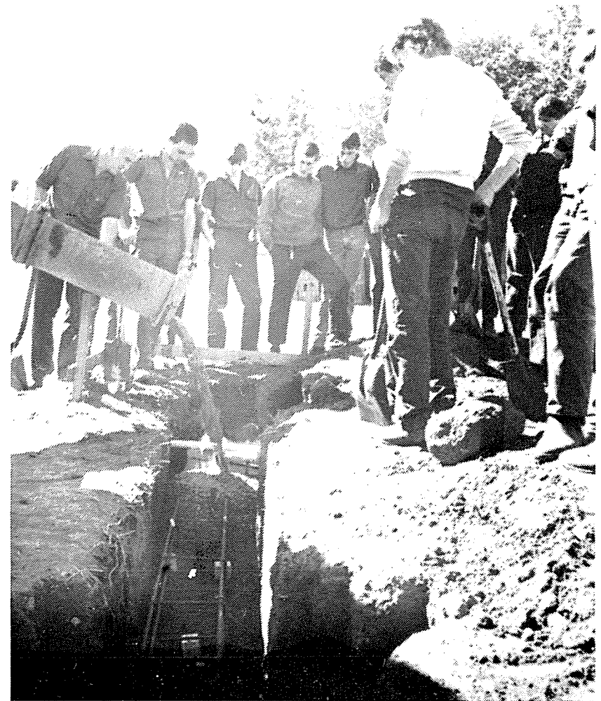
Footings for the new dairy.
